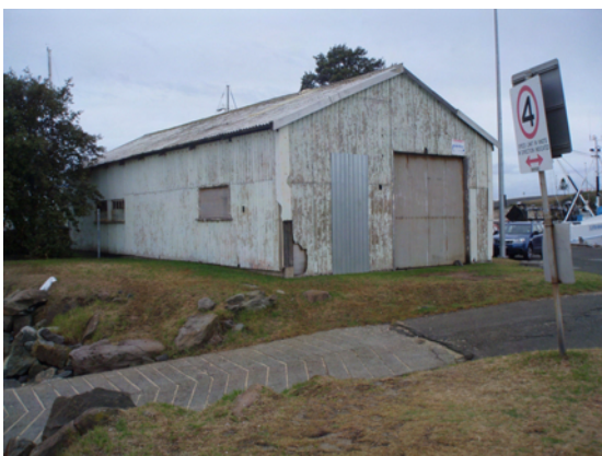
Poor condition of the existing work shed on the Central Pier.
